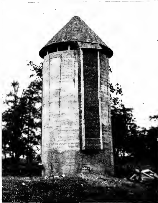
FIG. 208—THE WING CEMENT SILO.
